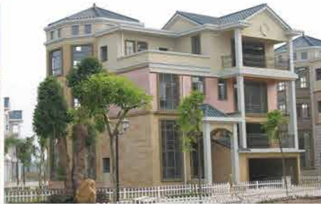
Wall Block in Villa
