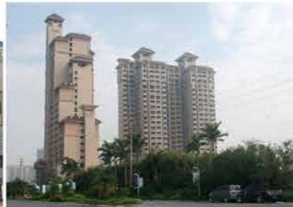
Wall Block in Condo
